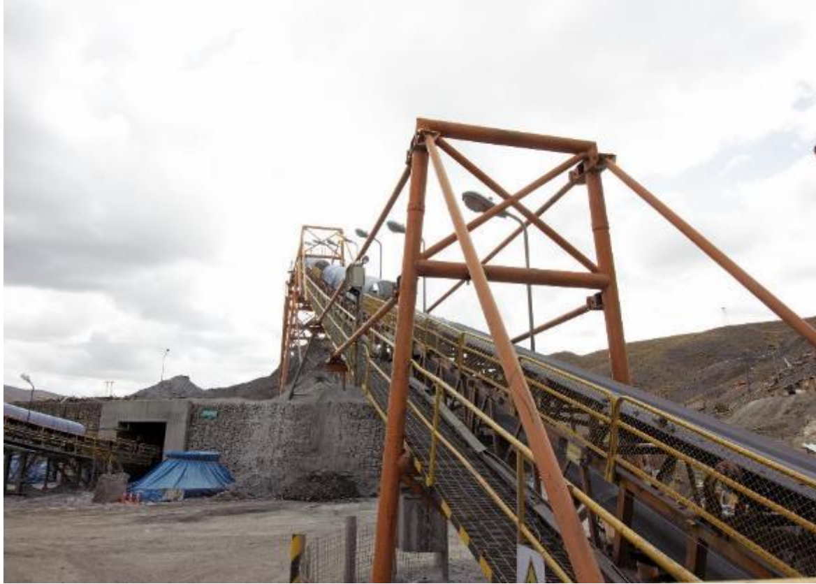
Conveyor and stockpile
